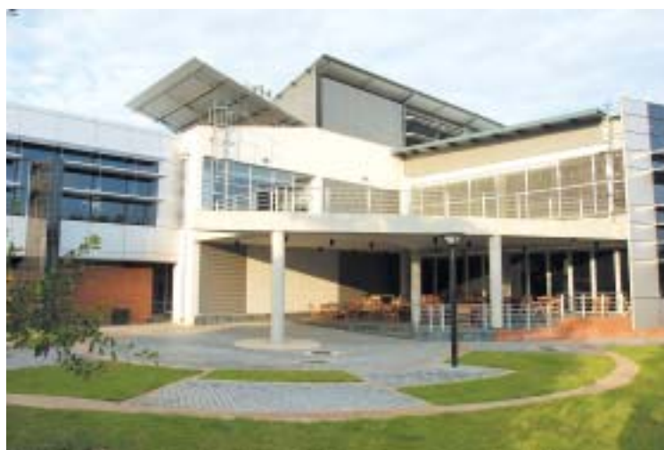
BOTEK's expertise in the design of energy efficient buildings is demonstrated in their own headquarters building.
