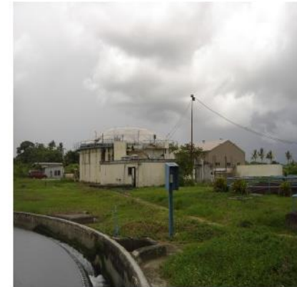
Anaerobic Sludge Digester
