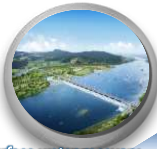
Surface water recovery
