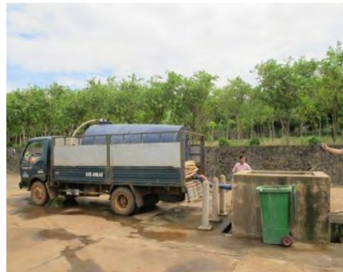
Co-treatment with wastewater at wastewater treatment plant
