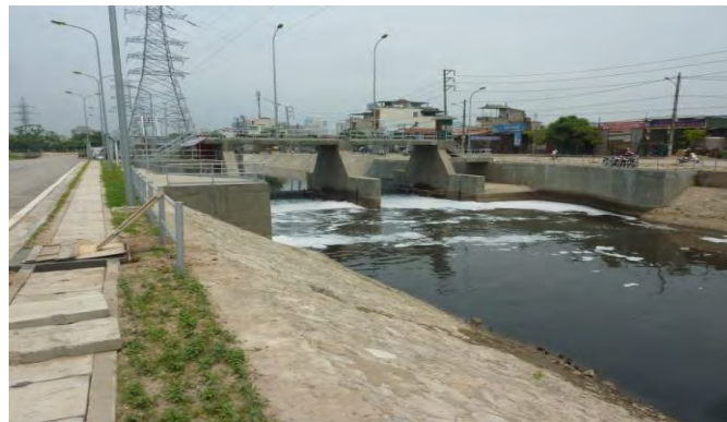
Figure 6: An open drainage canal is part of a combined sewerage and drainage system which has low organics and a low C/N ratio in wastewater coming into the wastewater treatment plant
