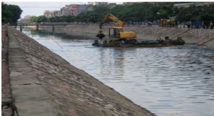
Figure 7: Sludge from combined sewerage and drainage systems produce high volumes and high levels of inorganic content.
