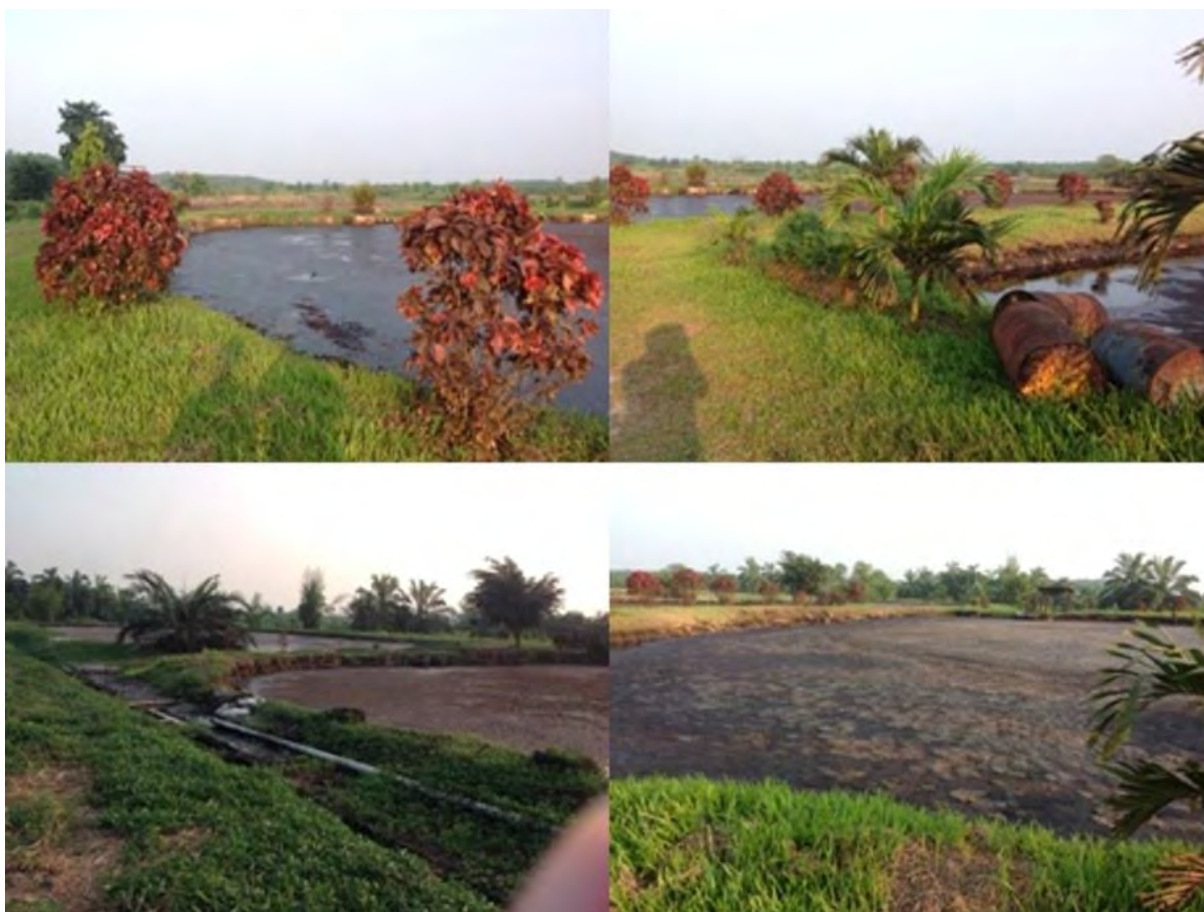
Figure 12: PTPN VI – rubber wastewater treatment
