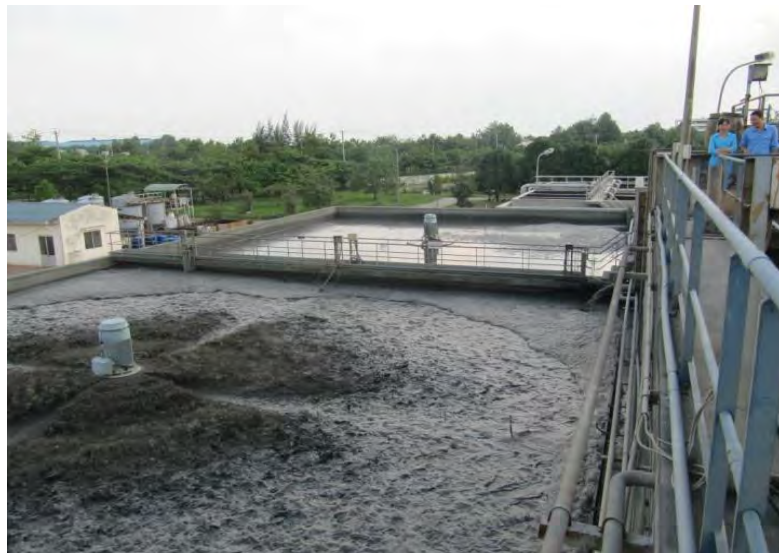
Figure 16: The biological wastewater treatment process requires certain start-up period
