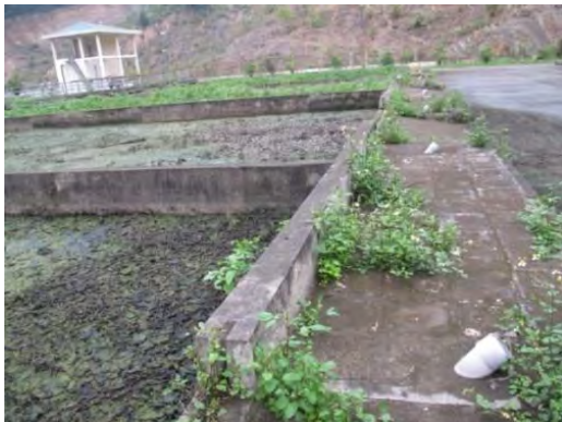
Sludge drying bed
