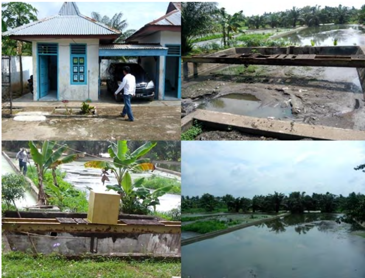
Figure 7: City sludge treatment plant in Jambi city
