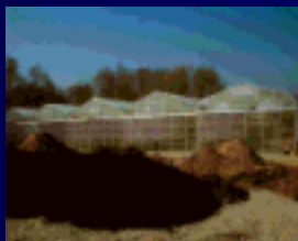
Solar drying of sewage sludge
