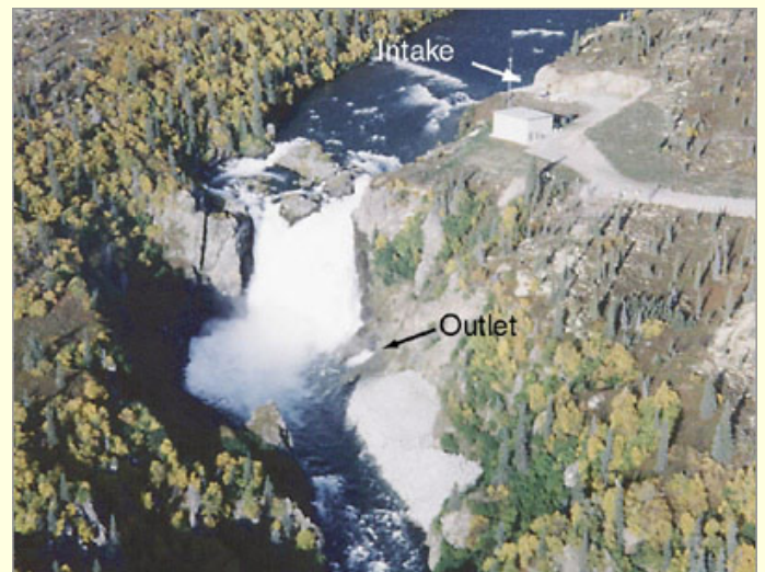
The Tazimina project in Alaska is a diversion hydropower plant. No dam was required.
