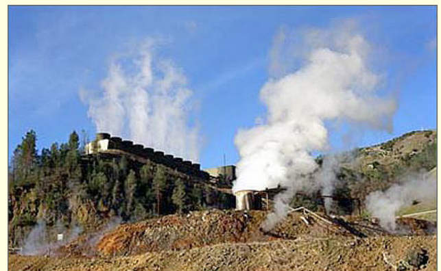
With a 750-MW output, The Geysers in California is the largest producer of geothermal electricity in the world. (Photo: David Parsons)
