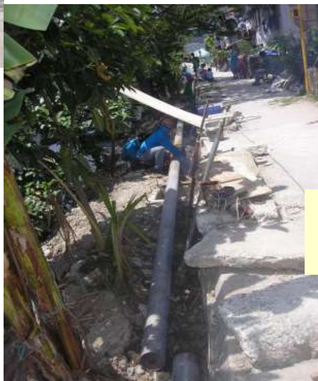
constructed wetland: gravel layer and outfall
