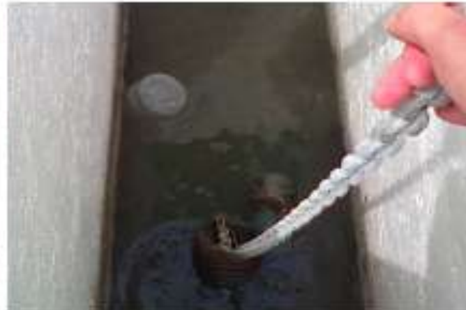
Flexible hose outlet for leak repair
