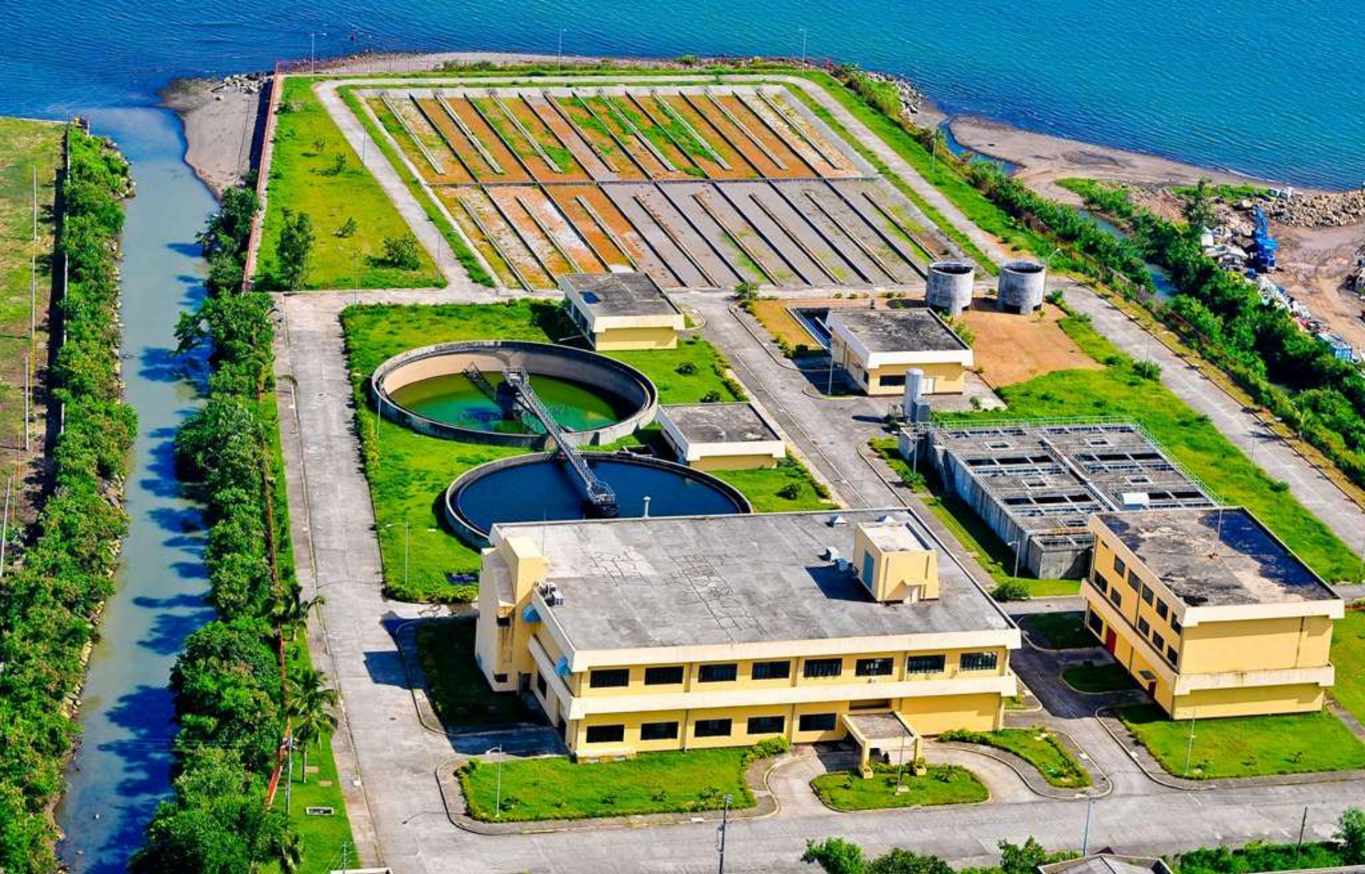
Wastewater Treatment Facility of the Authority of the Freeport Area of Bataan (AFAB) located in Mariveles, Bataan
