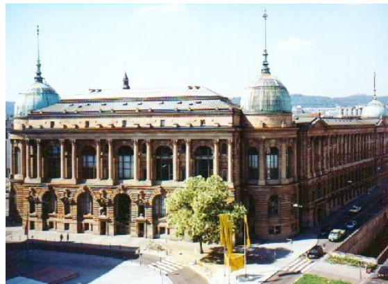
House of Business in Stuttgart - Headquarters' Location of the Steinbeis Foundation
