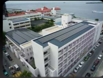
Hiriyaa School – 100kW
