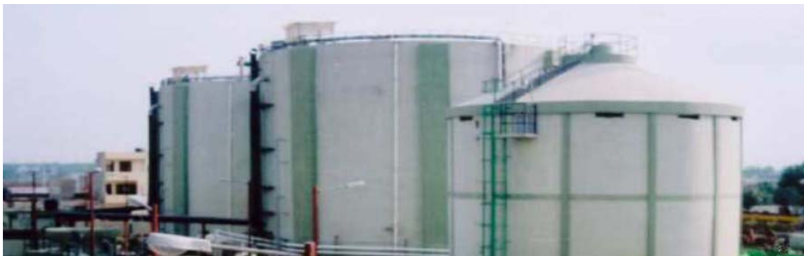
1.0 MW power project based on cattle dung at Haebowal Dairy Complex Ludhiana, Punjab
